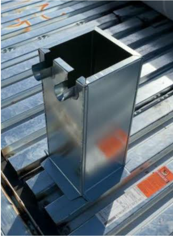
ENCLOSURE SHOWN IN PHOTO FOR REFERENCE ONLY - NOTE THAT ALL METAL MUST BE COATED METAL, (NOT GALVANIZED METAL)
