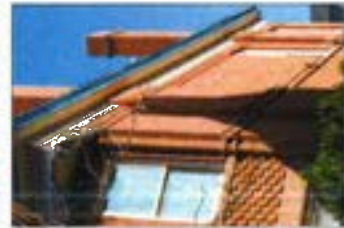
Brickwork lends itself to an endless variety of creative architectural compositions with essential elements like color and texture.
