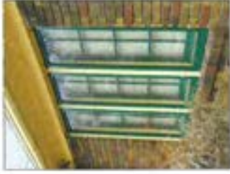
Exterior wood framed storm windows designed to fit the primary framework of the original.
