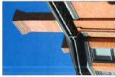
Attention to the brick texture and the pointing profile are used in this case to define the wall, the window bay and the chimney.
