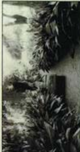
The garden walls constructed during the 1920s and 1930s at Shadow-on-the-Tribe in New Haven, Louisiana, also help to define the historic landscape. As part of the restoration project, the creator used a mixture of earth and Portland cement to reconstruct the walls and new stone (locally found), a gravel top coat is placed and called for (book cover and called for book) (Shadow-on-the-Tribe)
