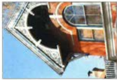
Using non-pairable substitute materials may preclude enhancing architectural details through a carefully considered color scheme.
