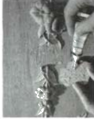
In Preservation, an appropriate level of intervention is established prior to work in order to maximize retention of historic materials. (A) A conservator is applying adhesive to 19th century composition ornament that has delaminated from its wood substrate. (B) The composite fragment is carefully held in place until the quick-setting adhesive takes hold. Photos: Jonathan Thomson.
