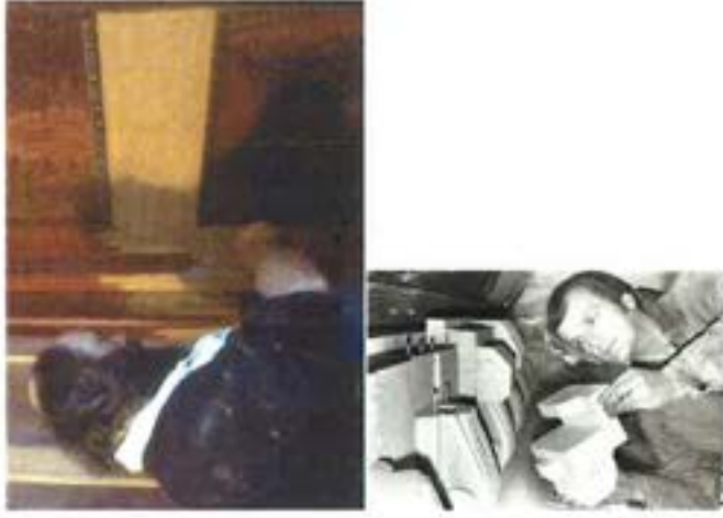
Figures 2-17 and 2-18. Skilled craftsmen from across the U.S. were employed in the Kearns Mansion restoration of the late 1970s. Credit: Arrington & Swinton.
