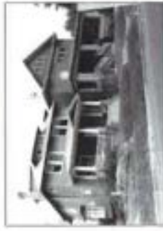
Because of its simplicity, the Foursquare lends itself to many styles. With thick square posts and exposed rafters it takes on a Craftsman tone. Wide rounded porch columns and a pediment on the porch roof, it becomes Colonial.
