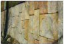
Natural stone paving and landscaping enrich the streetscape.
