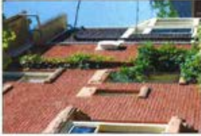
A new addition which is subordinate to the house and distinguished by height, materials, foundation and unique profiles and details.
