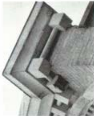
Two examples of "limited replacement in kind" show an appropriate scope of work within the treatment. Preservation. (a) One metal installation that has sustained damage from a faulty gasket will need to be replaced, and (b), neglected repairs to deteriorated wood cornice element (fauxon board and wood lions) mean that most of the historic materials were retained in the work.
