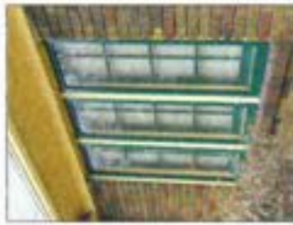
Central wood storm windows designed to fit the primary framework of the original.
