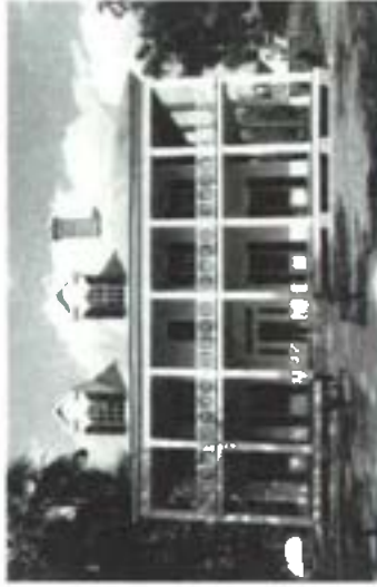
The Brown-Mulholland House in Tallahassee, Florida, in 1895, is shown (a) before and (b) after the restoration. Over the years the east (far right) side of the veranda had been jilted in a acid-bay. During the restoration, the floor joist was removed and the east veranda, together with its flooring, stairs, and foundation, restored. Photo: City of Tallahassee, Community Development Department.
