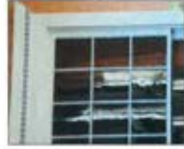
The reflective ripple characteristics of curly glass can be appreciable when compared to the regular surface of more recent replacement glass.
