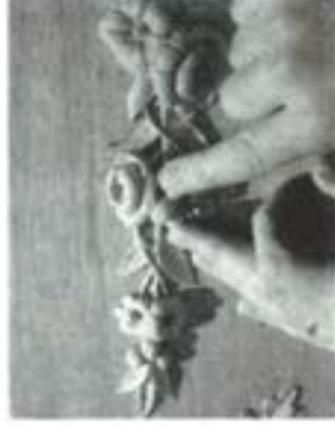
In Preservation, an appropriate level of intervention is established prior to work in order to maximize retention of historic materials. (A) A conservator is applying adhesive to 19th century composition ornament that has delaminated from its wood substrate. (B) The composite fragment is carefully held in place until the quick-setting adhesive takes hold. Photos: Jonathan Thomson.
