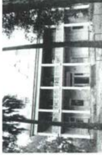
The Brown-Mulholland House in Tallahassee, Florida, in 1895, is shown (a) before and (b) after the restoration. Over the years the east (far right) side of the veranda had been jilted in a acid-bay. During the restoration, the floor joist was removed and the east veranda, together with its flooring, stairs, and foundation, restored. Photo: City of Tallahassee, Community Development Department.
