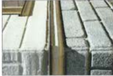
Masonry and weathered stonework here combined with a new concrete profile, demonstrating a mix of architectural time and history.
