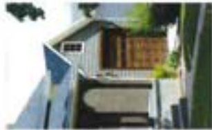
Recent, two-level garage addition designed to match main structure
