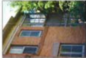
Early rear addition following the tradition of continuing the roof line, sloping back and using contrasting materials and fenestration.
