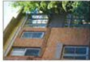
Early rear addition following the tradition of maintaining the main line, supporting deck and using mismatching materials and finishes.
