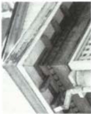
Two examples of "limited replacement in kind" show an appropriate scope of work within the treatment. Preservation. (a) One metal installation that has sustained damage from a faulty gasket will need to be replaced, and (b), neglected repairs to deteriorated wood cornice element (fauxon board and wood lions) mean that most of the historic materials were retained in the work.
