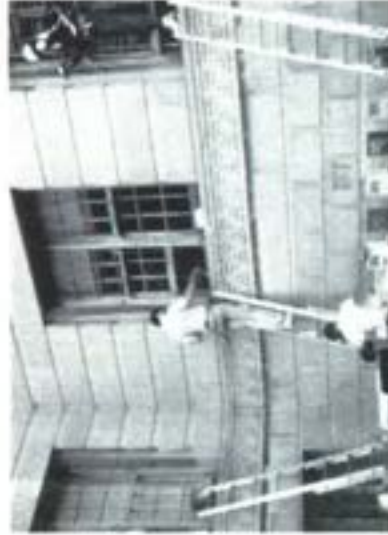
Preserving a building's historic windows generally involves cleaning, sanding, and repainting. While some repair work will most likely be undertaken within the scope of work on the institutional building, replacement of the window units will usually not be an appropriate preservation treatment. Photo: Chuck Fisher.
