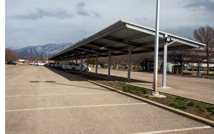
Above: Tools used at the DWR Mantua Fish Hatchery Building. Below: Solar Parking Array at the Taylorsville State Office Building
